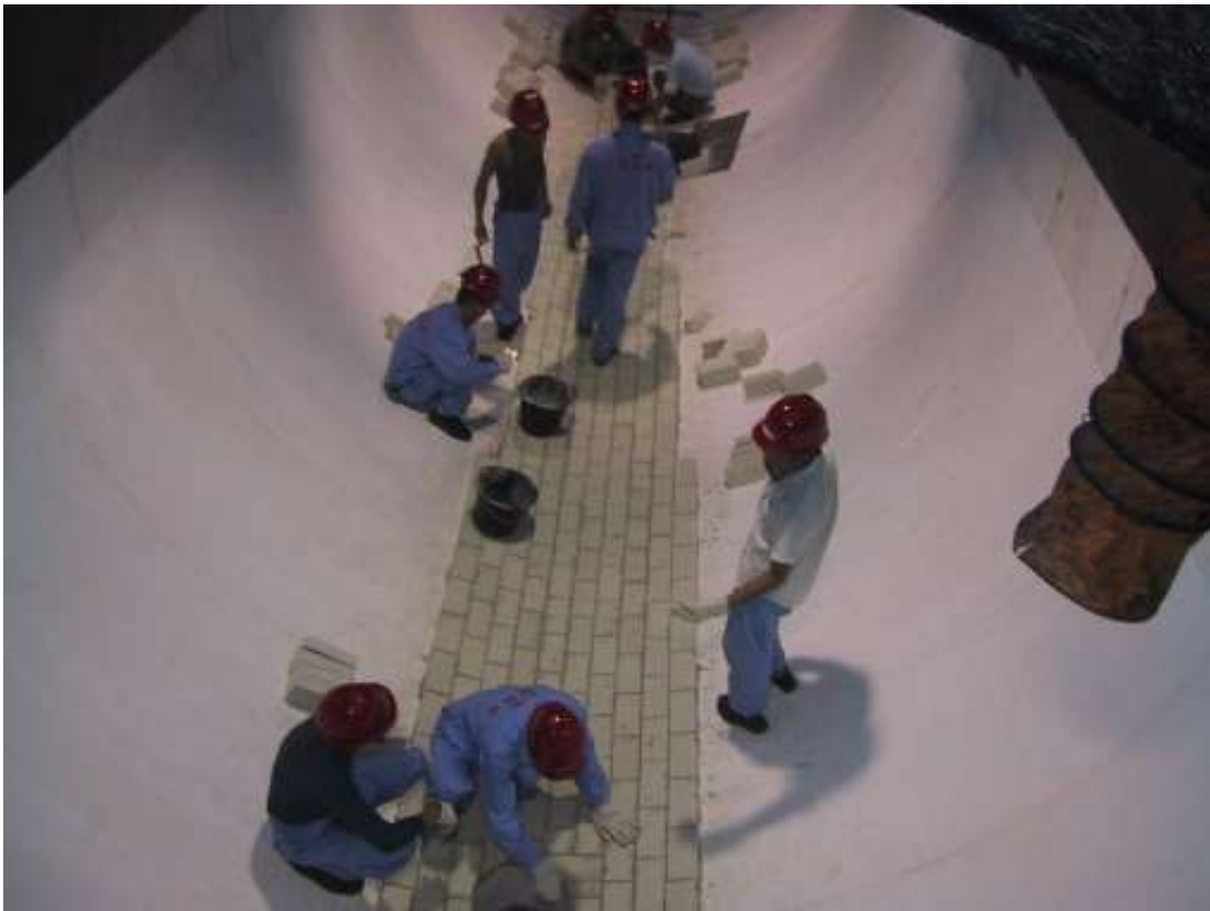
Image 3: Beginning of brick lining on top of the membrane.
