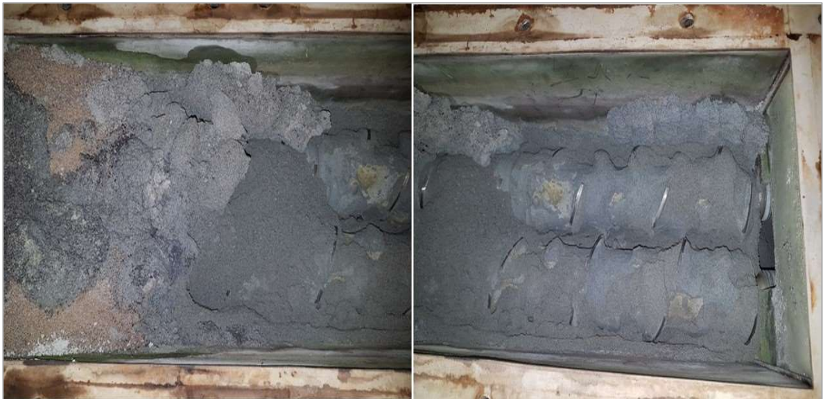
Figure 13: Pug Mill Interior After Shutdown
