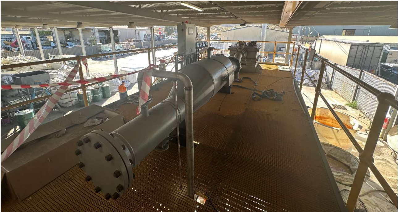
Figure 8: Sulphur condenser for kiln offgas
