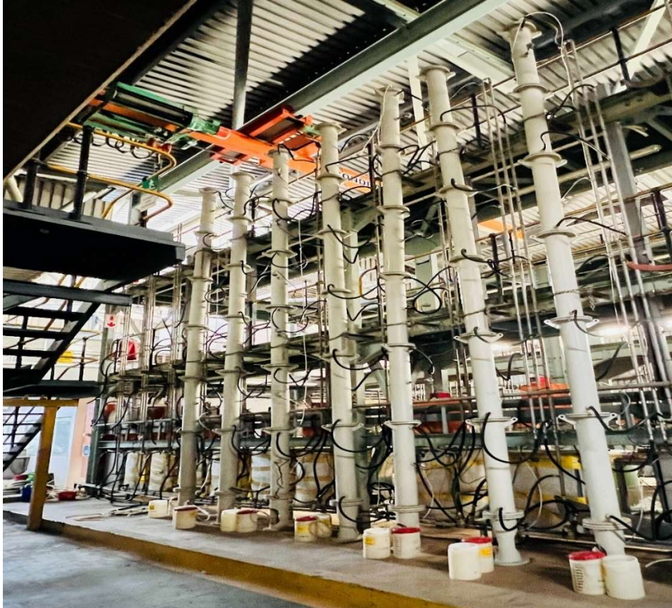
Figure 1: 6 m Column Set-up
