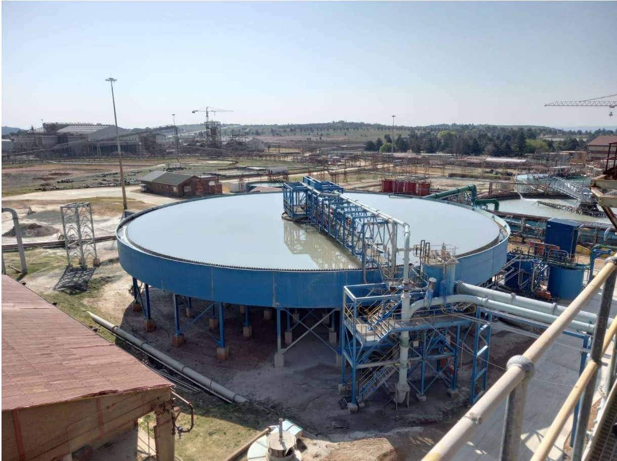
Figure 11: DRD Gold's Ø45 m thickener.
