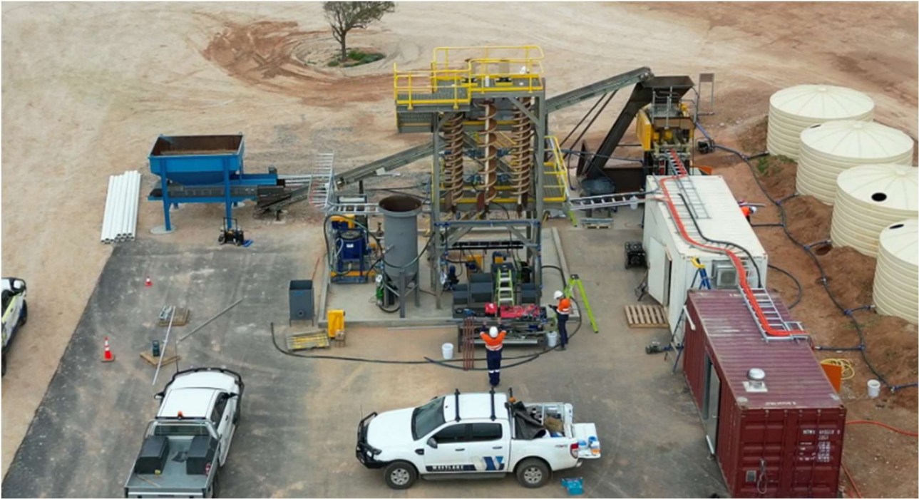
Figure 4: Demonstration Plant concentrator during construction
