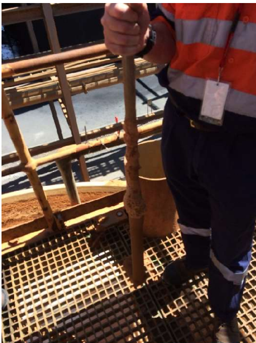
a) Probe/rod that scale grows on
