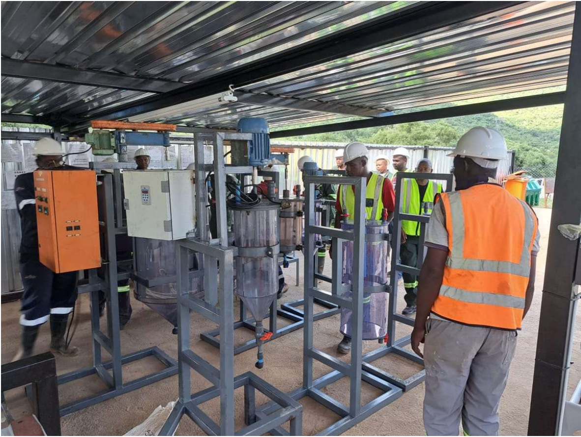
Figure 17: Plant being installed.
