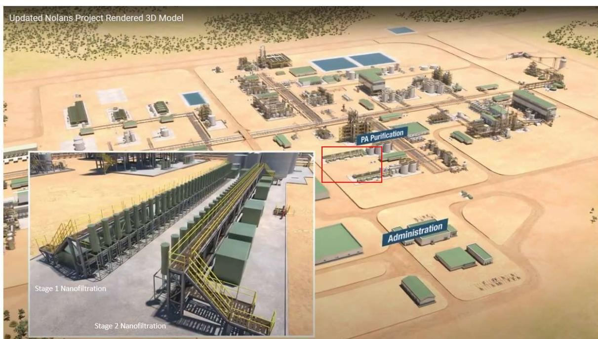
**Figure 7 – PA Purification Circuit at Nolans Hydrometallurgical Processing Facility <sup>7</sup>**
