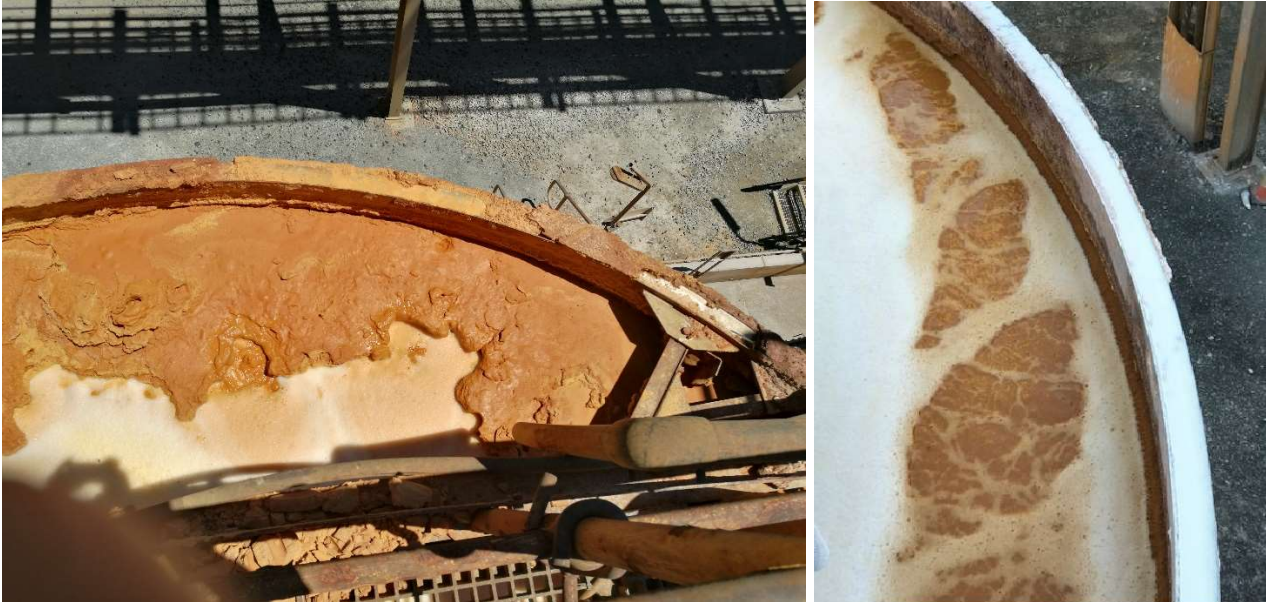
a) Typical scale in conventional tank
