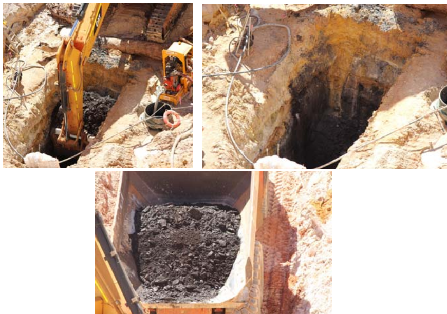
Ambassador East – Excavation of Bulk Ore sample #1 for Piloting (17 th February 2016)
