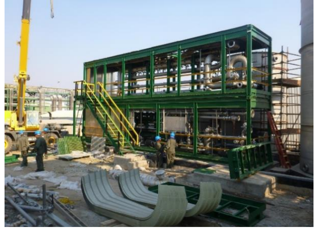
Skid installation completed within weeks
