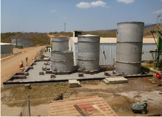
Pad installed while Skids being fabricated
