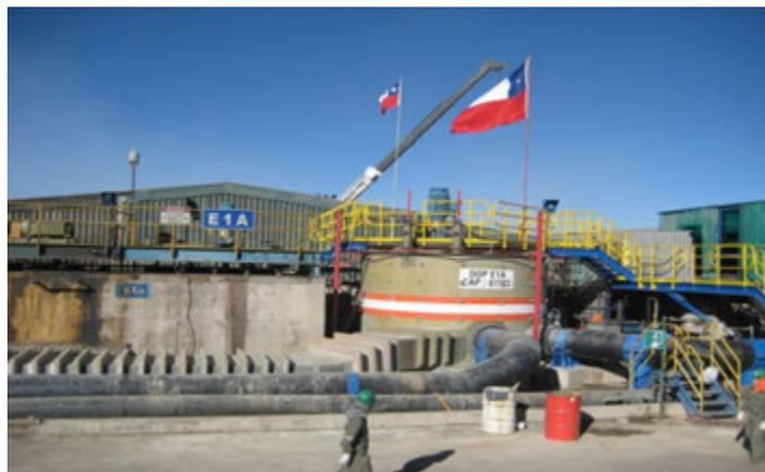
**Picture 2:** E1 stage of Chuquicamata Oxide Plant Train A after the retrofit project (the new DOP<sup>®</sup> pump at the front).
