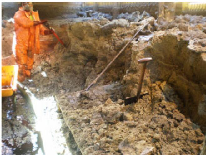
**Picture 1:** E1 settler of Outotec reference plant being cleaned of precipitated gypsum. Prior to the maintenance shutdown, the plant was operated with >1 m thick gypsum layers in the settlers.
