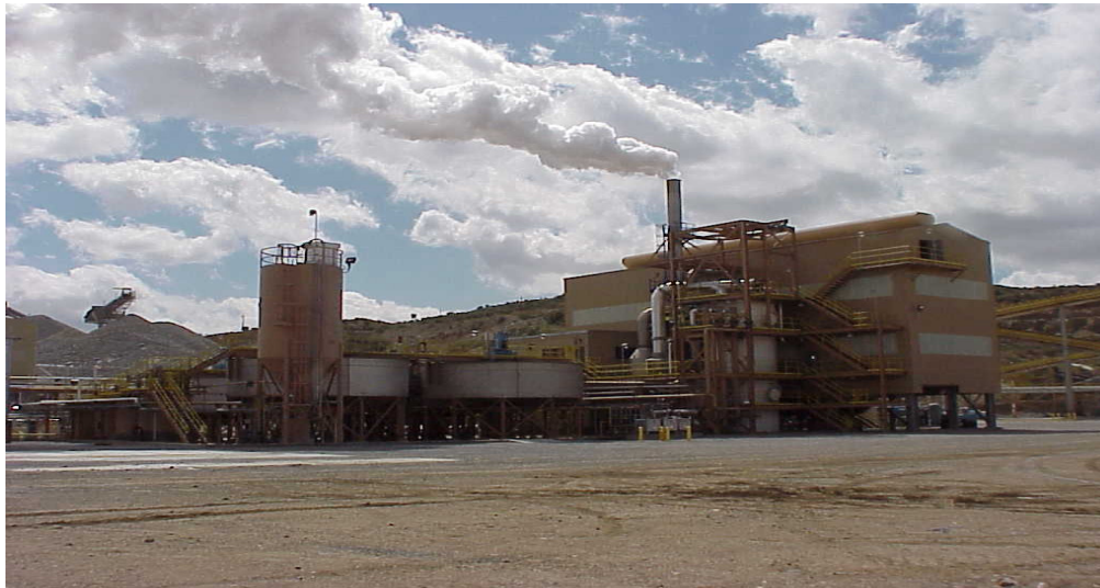
Phelps Dodge Pressure Oxidation Demonstration Plant
