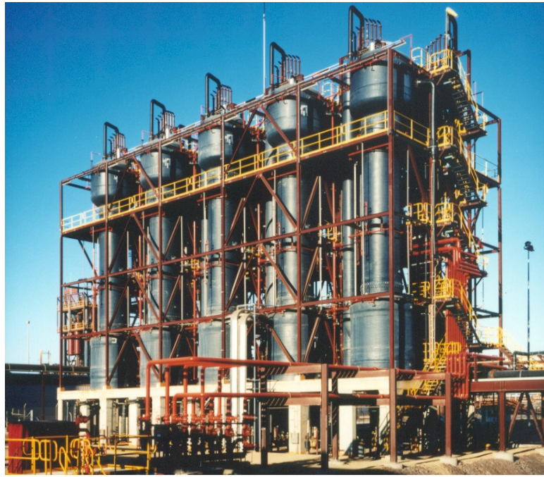
Fig. 6 Bateman Pulsed Column Installation at Olympic Dam
